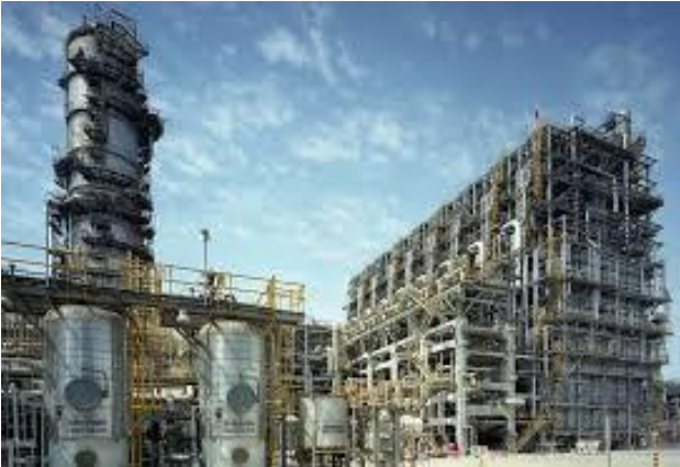
Biskra & Jijel 1600MW Power Plant Project – Algeria
